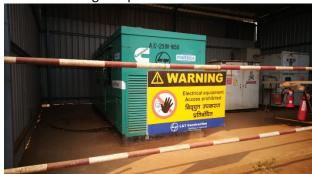
v. The gaseous emissions from DG set shall be dispersed through adequate stack height as per CPCB standards. Acoustic enclosure shall be provided to the DG sets to mitigate the noise pollution. Low sulphur diesel shall be used. The location of the DG set and exhaust pipe height shall be as per the provisions of the Central Pollution Control Board (CPCB) norms.
