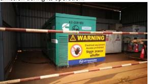
v. The gaseous emissions from DG set shall be dispersed through adequate stack height as per CPCB standards. Acoustic enclosure shall be provided to the DG sets to mitigate the noise pollution. Low sulphur diesel shall be used. The location of the DG set and exhaust pipe height shall be as per the provisions of the Central Pollution Control Board (CPCB) norms.
